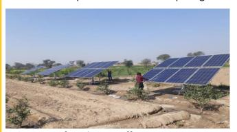
system was found more efficient, energy saving, economical and environmentally safe as compared to diesel operated drip irrigation system, even though its initial installation cost is very high. It was also found that the solar system is more economical in terms of operation therefore, it is recommended to install solar panels for pumping units.
